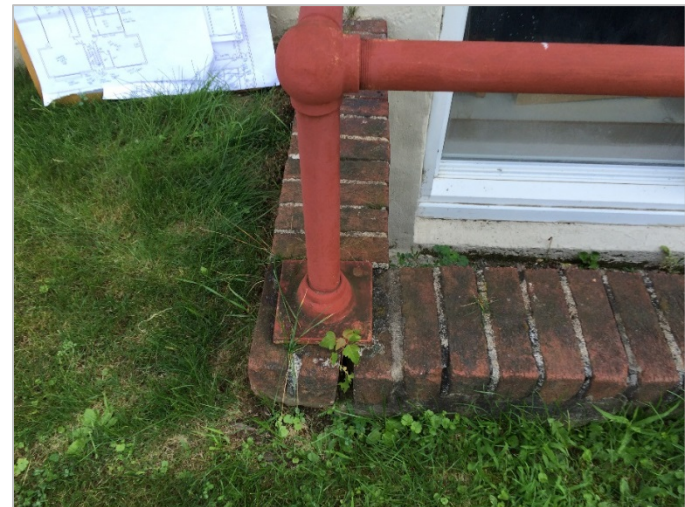
Port Dickinson masonry restoration
