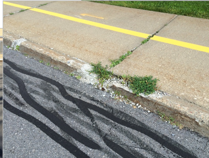
Port Dickinson bus loop sidewalk
