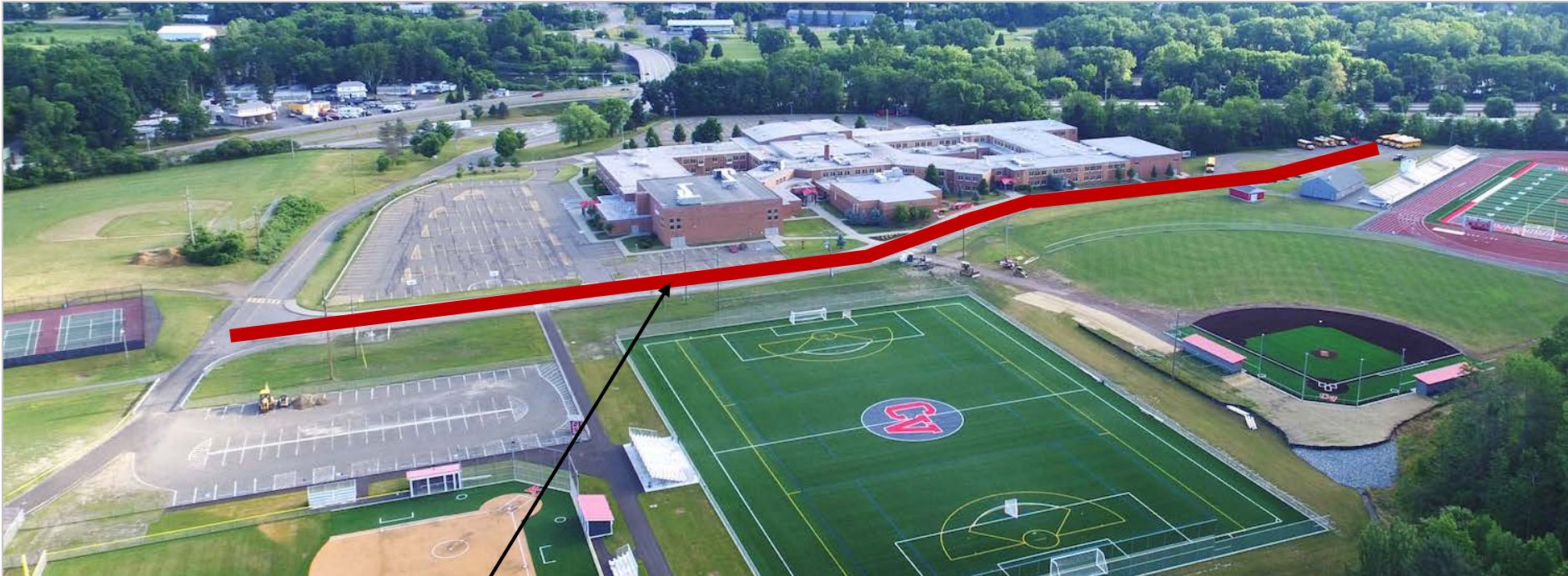
Location of pavement reconstruction
