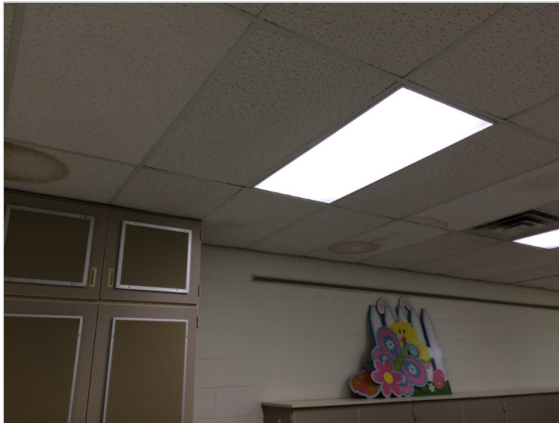
Chenango Bridge fluorescent lights
