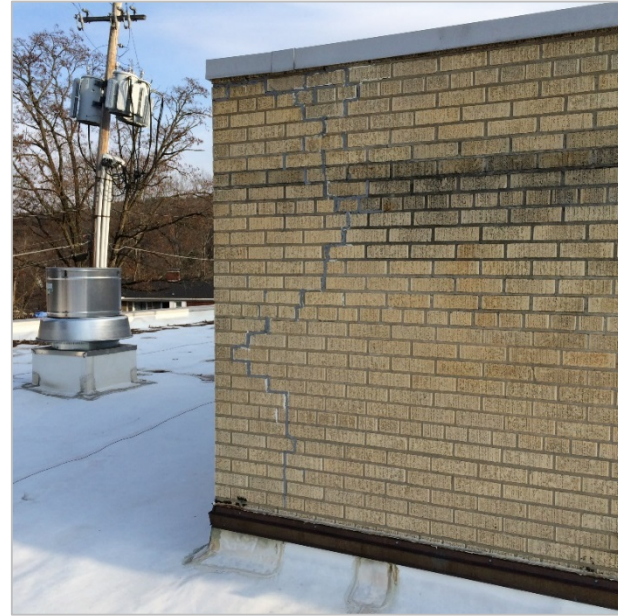
Chenango Bridge masonry restoration
