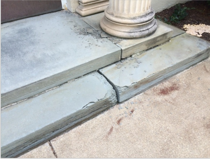
Port Dickinson original entry stair deterioration
