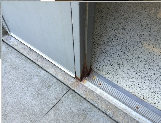
Middle School / High School doors
