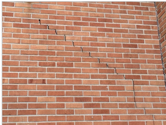
Middle School / High School masonry restoration
