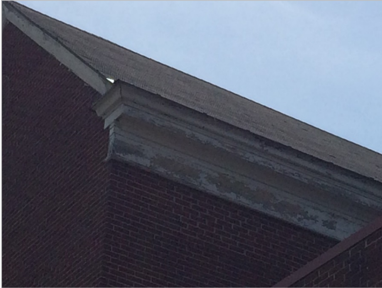
Wood trim deterioration
